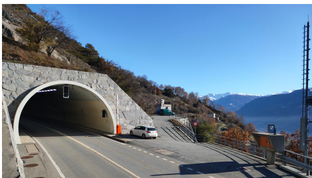
Tunnel Mittal Goppenstein
